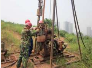
SPT&amp;CPT Geological Exploration
