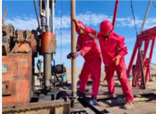
Wireline Diamond Core Drilling
