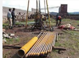
Subgrade Grouting Hole Drilling
