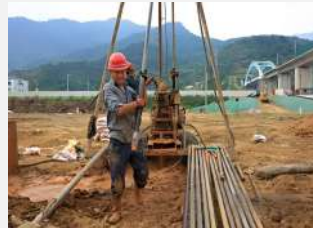
Concrete Inspection Hole Drilling
